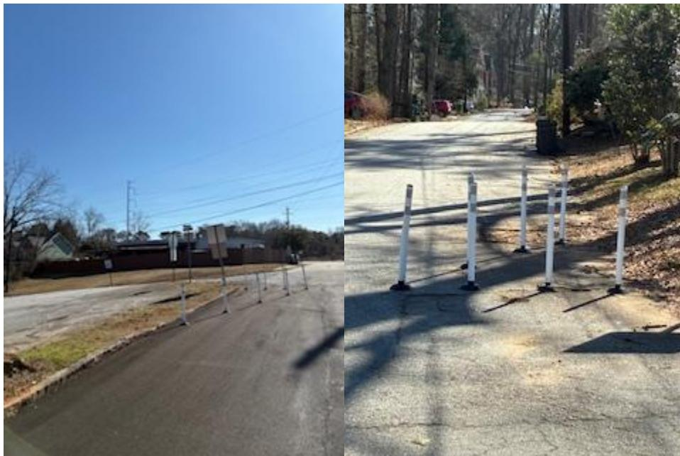
Right of Way obstructions were removed at the corners of Spruce Drive and Lakeshore Drive and Spring Drive and Poplar Road. The two hardened structures were removed to increase traffic safety. The two structures were replaced with reflective traffic delineators.
